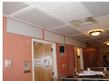
FIG. 5. Sound absorbing panels installed on the hallway ceiling and walls.
