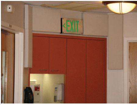
FIG. 6. Sound absorbing panels installed around a corner cabinet.
