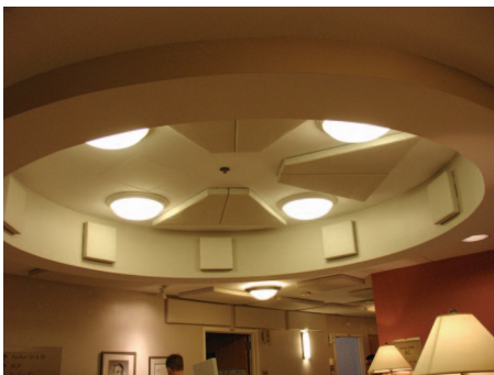
FIG. 7. Sound absorbing panel treatment of a large circular architectural feature at the nurses's station. Note a person shown at the bottom center for scale.
